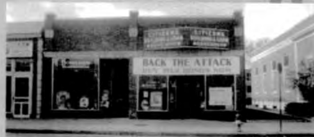
WWII PATRIOTISM. 8406-08 Georgia Avenue as it looked in 1943. "Back the Attack" was a WWII victory exhibit sponsored by The Washington Post and held on the grounds of the Washington Monument. The sign in the window of Frank L. Hewitt's Citizens Building & Loan Association features a quote by General Dwight D. Eisenhower that reads "We are playing in the big leagues. You can't hit a home run by bunting. You have to step up there and take your cut at the ball." The analogy referred to the all-out Allied invasion of Italy on September 3, 1943, rather than individual attacks on "stepping stones" such as Sardinia, Corsica, or Crete. PHOTO BY NELLE HEWITT PHOTOGRAPHY
