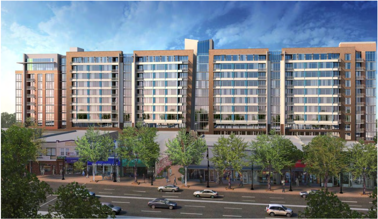
Georgia Avenue elevation, looking east
