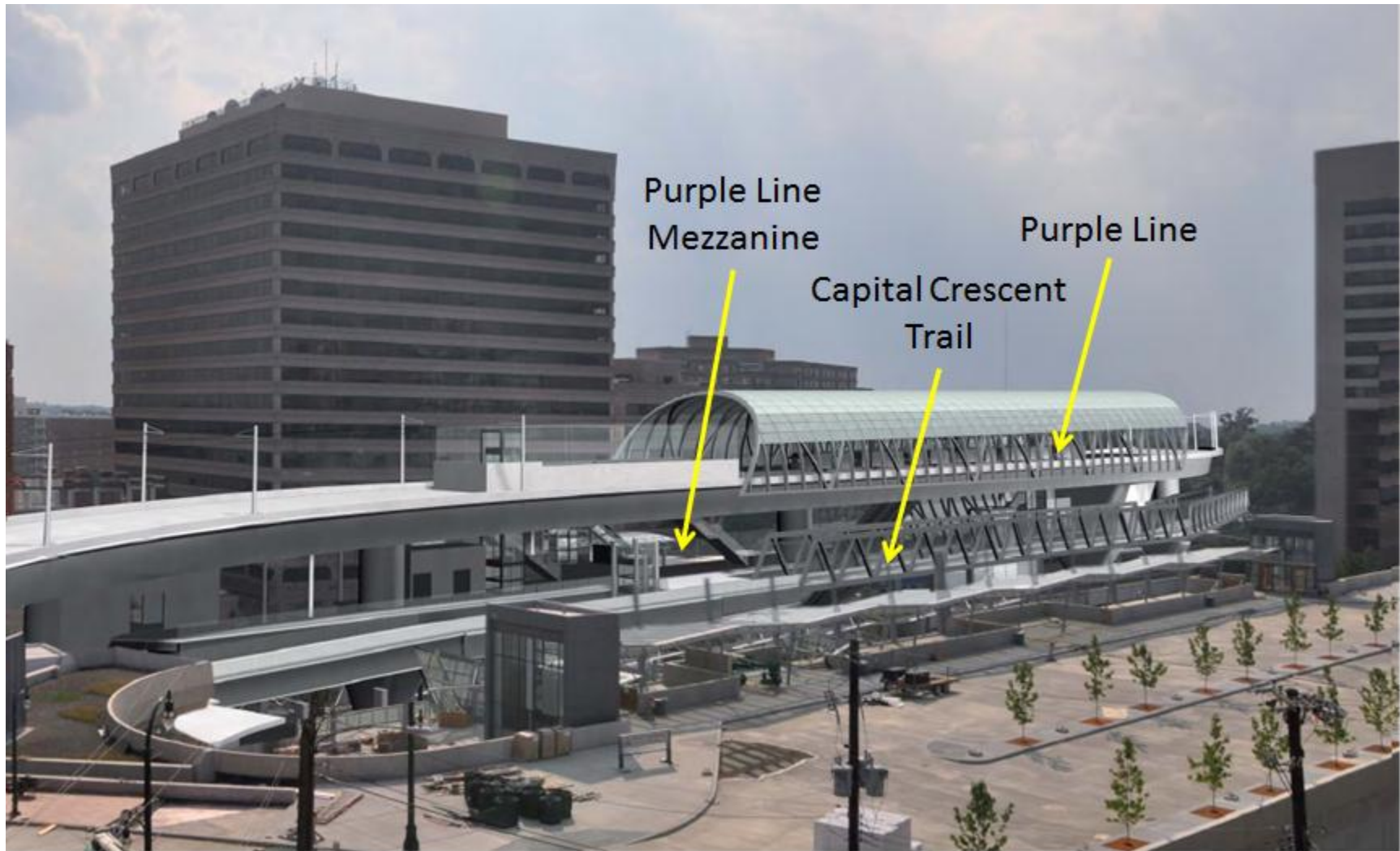
A rendering of the Silver Spring Transit Center area looking toward the Purple Line and Red Line from Bonifant Road.
