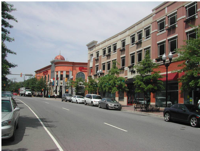
Punched window openings with planters give this parking garage the illusion of enclosed interior space
