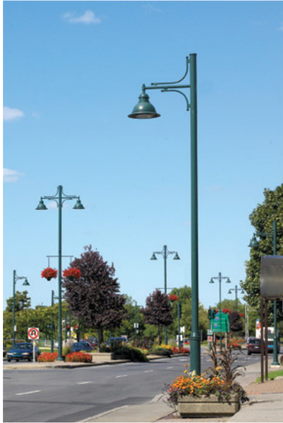
Street lighting: Spring City Washington series in Federal Green or approved other
