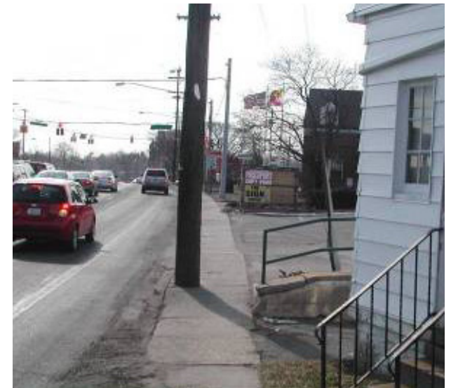
Existing condition: Obstructions and the proximity of traffic make this sidewalk along Connecticut Avenue unsafe
