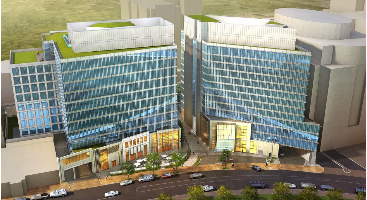
Image of the hotel and office buildings from Woodmont Avenue
