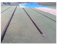
underlying soil did not percolate well. 2-inch drain pipes were installed at 18-inch depths on 6-foot centers throughout the greens. These projects will have a very positive impact on playability, but the big win is for the environment, since these "problem" greens often required extra plant protectants (especially fungicides), and required a lot more cultural practices and large fans (using a lot of fuel) to help dry them out. More information on MCG blog here: http://bit.ly/Wg9szD.
