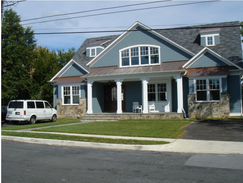
Front view of existing building from West Virginia Avenue
