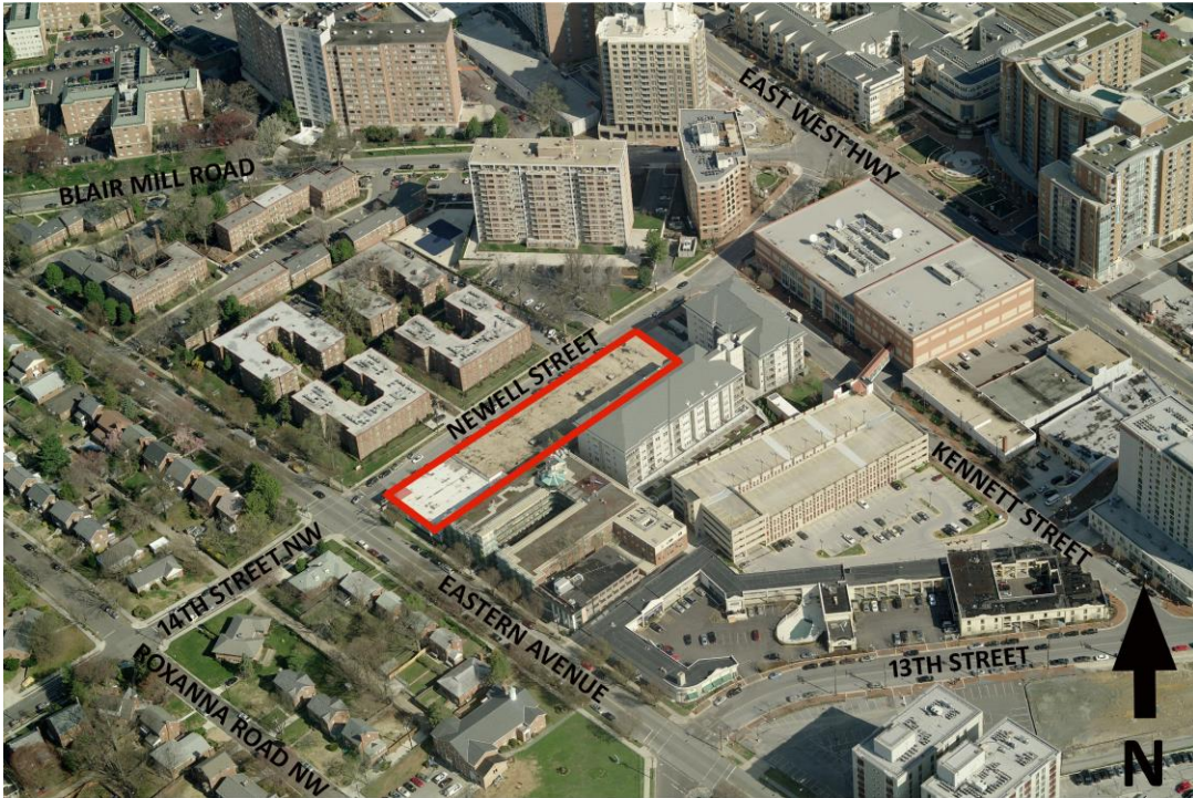
Aerial Photo Looking North
