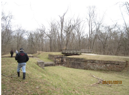
Figure 4: Broad Run Trunk, C&O Canal
