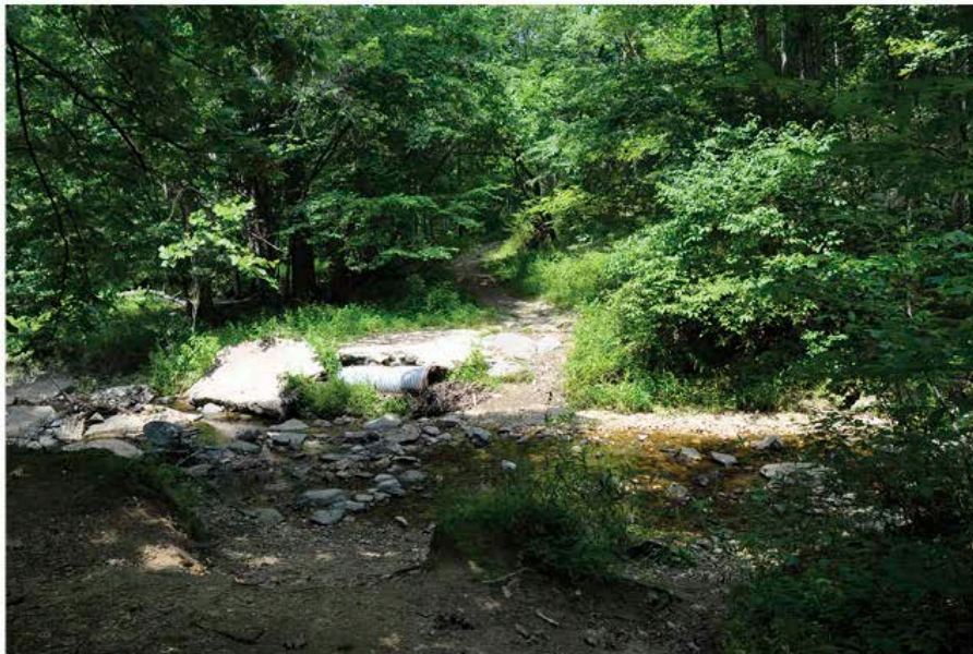
Figure 13 – Stream crossing of a tributary to the North Branch. Concrete and pipes will be removed and replaced with either a bridge or boardwalk.
