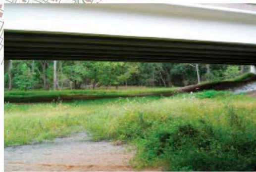
Existing Condition under ICC
