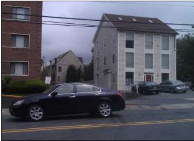
Three story office building as seen from Battery Lane
