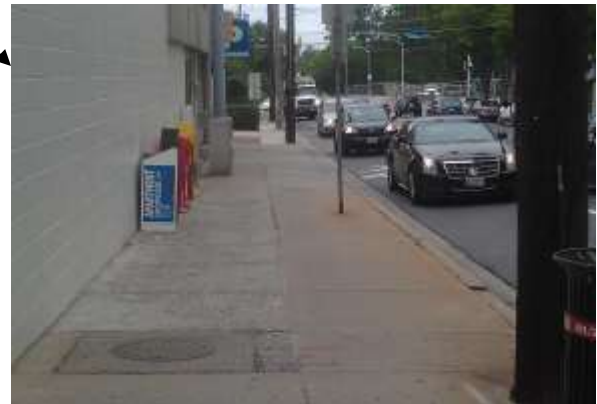
Adequate sidewalks exists along Woodmont Avenue
