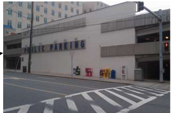
Woodmont Avenue/ Rugby Ave. Public Parking Garage
