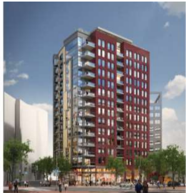
Approach from Edgemoor Lane
