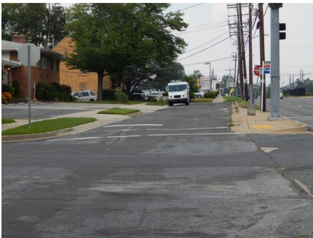
Figure 5: New Hampshire Avenue Service Road (@ signaled intersection)
