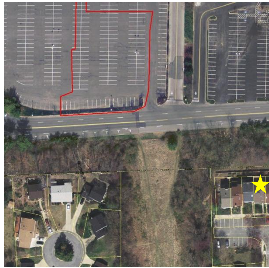
Figure 29 Adjacent properties with the greatest impacts
