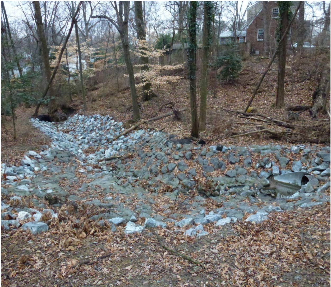
Westfield's stormwater outfall into Silver Creek
