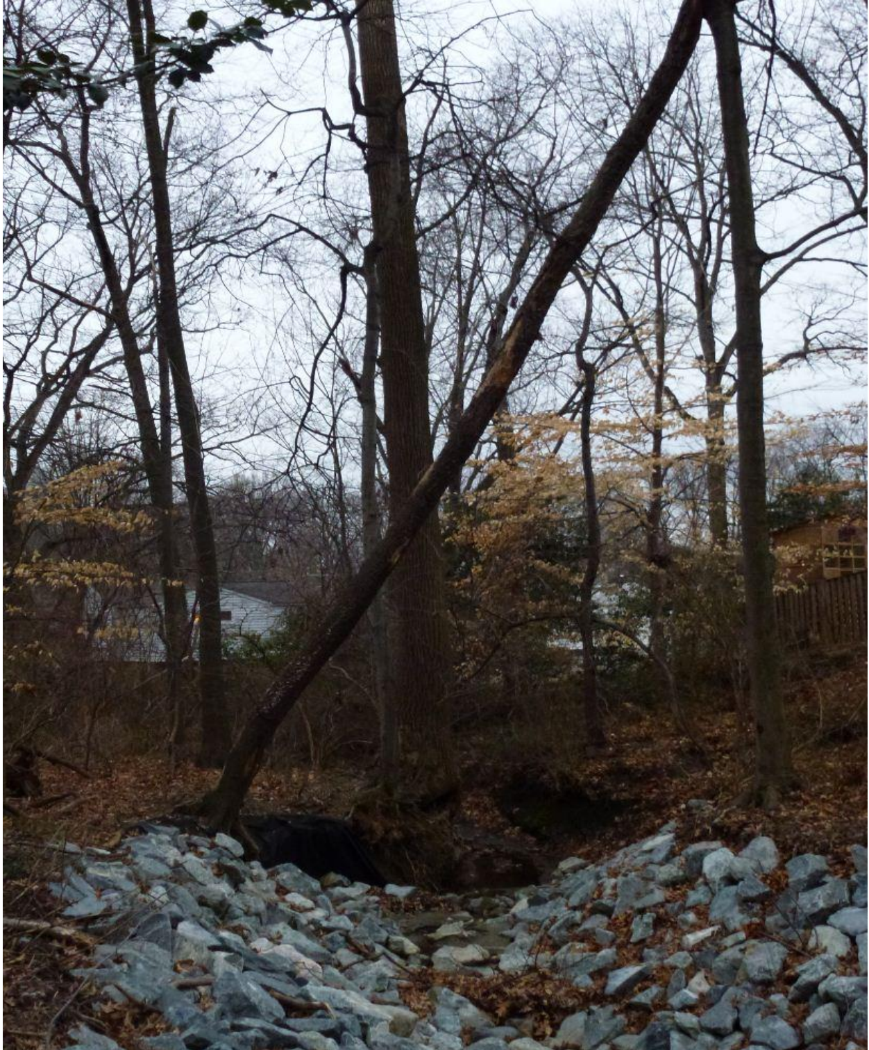
Stream bed and critical root zone damage
