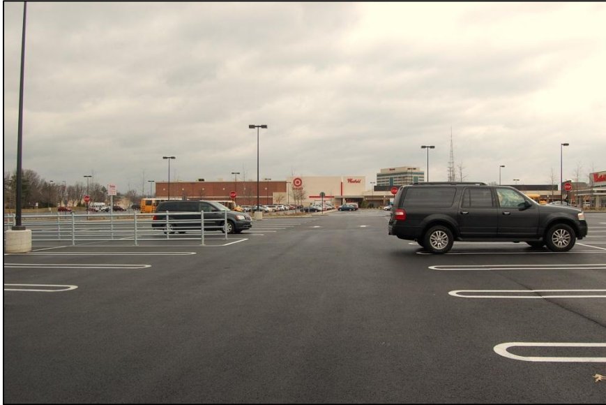
Figure 1: Westfield Wheaton Parking Lot, looking north
