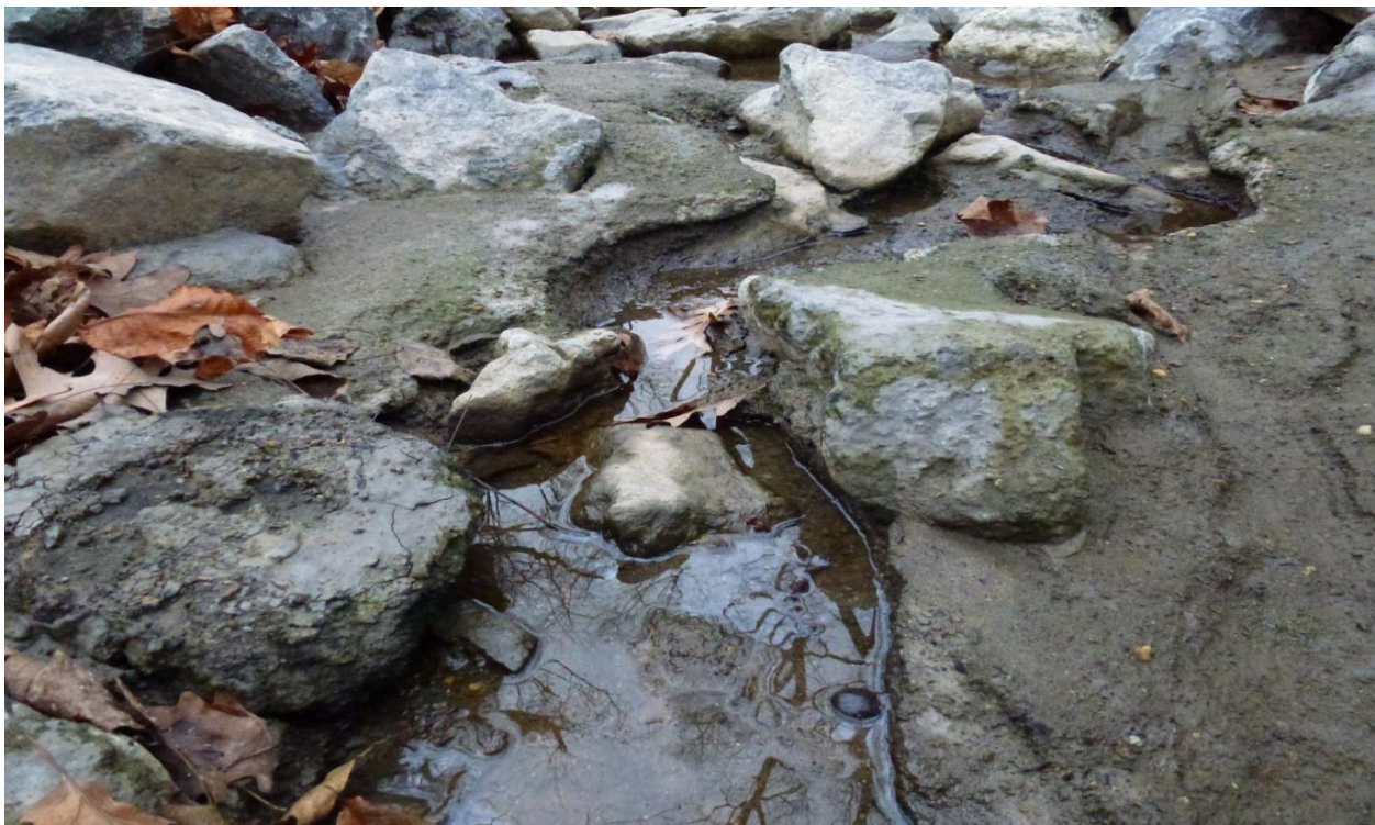
Stormwater gouging a new erosion gully in the concrete seal
