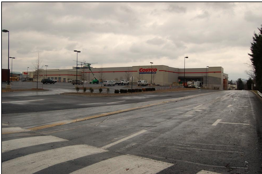
Figure 3: Westfield Wheaton Parking Lot, looking east
