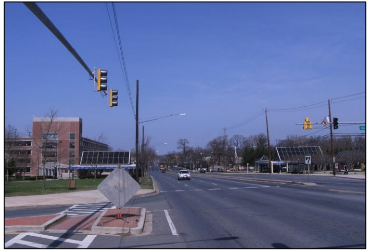
Existing Condition: The newly constructed Metro garage along Georgia Avenue is approximately 82' feet tall
