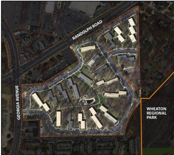
The hiker/biker connection would provide an important link from the Glenmont Core
