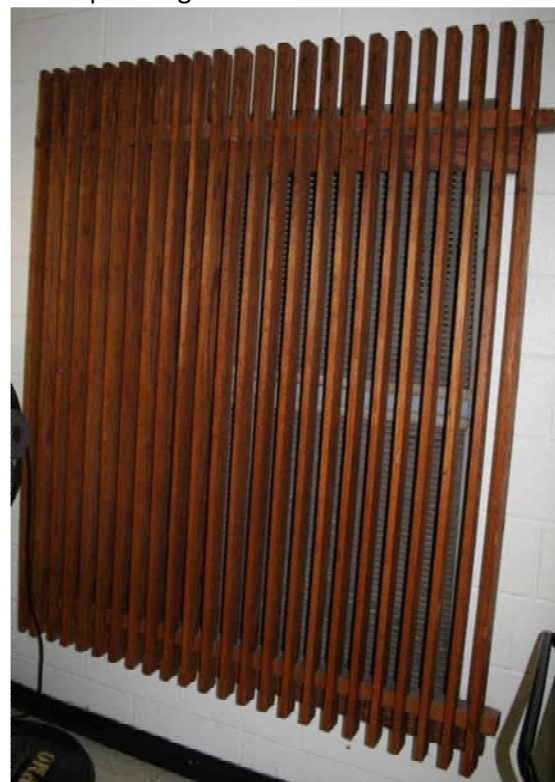
F: Wood screen as built, in activity wing hallway
