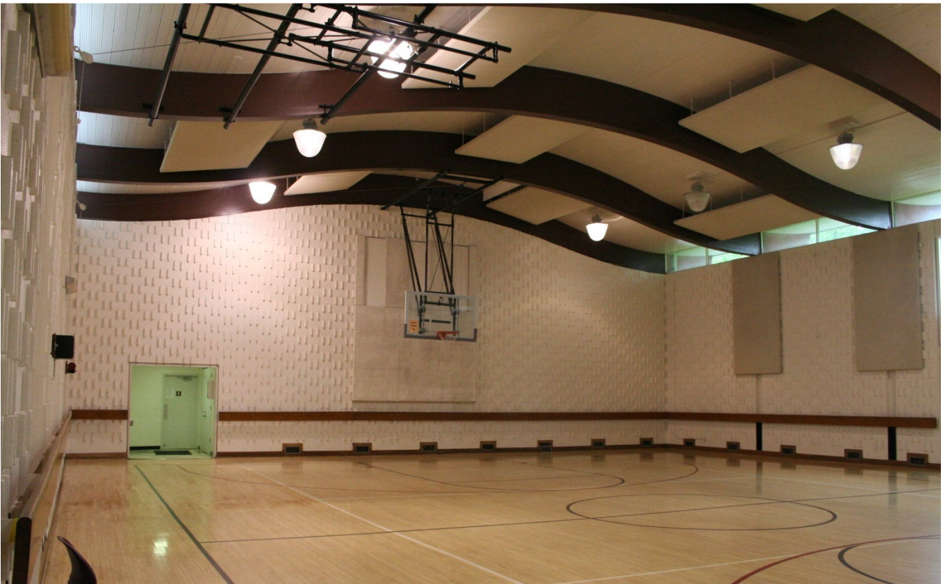
FIGURE 14: The massive, curved beams are exposed in the auditorium interior. Glass panes at the top of walls not only bring in natural light but enable one to see the entire form of the graceful arched supports. (Clare Lise Kelly, June 2013)
