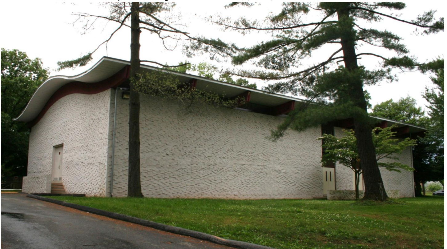
FIGURE 13: Northeast Corner, Auditorium. (Clare Lise Kelly, 6-2013)
