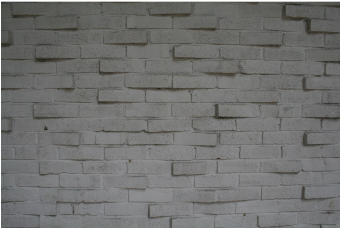
A: Masonry texture: brick walls of the activity wing
