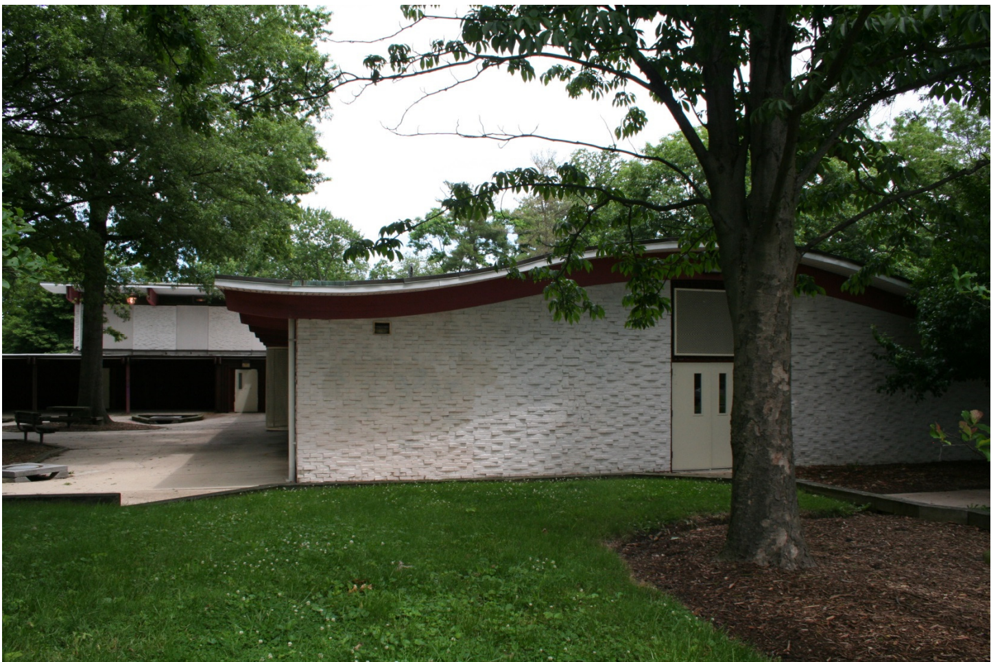
FIGURE 10: South Elevation. (Clare Lise Kelly, June 2013)
