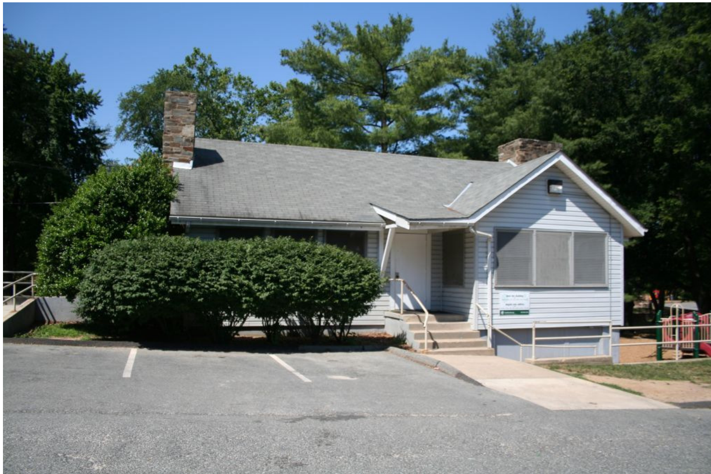
Figure 9. Pinecrest Recreation Building, front (north) façade.
