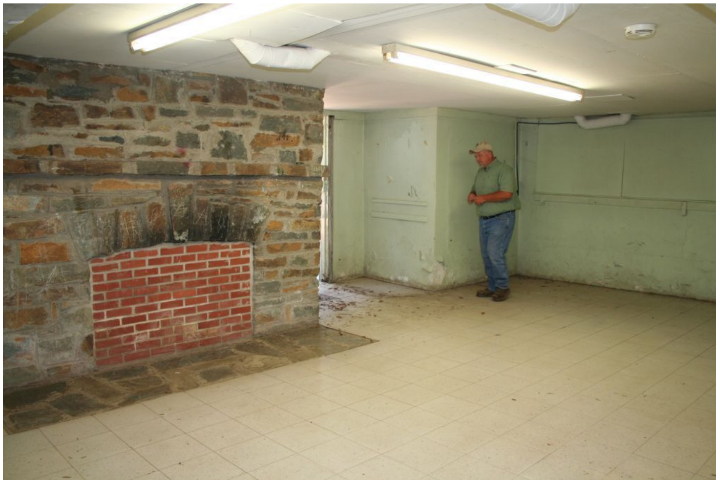
Figure 15. Interior detail of hearth, fireplace (bricked in), and mantle in the basement floor of the Pinecrest Recreation Building.
