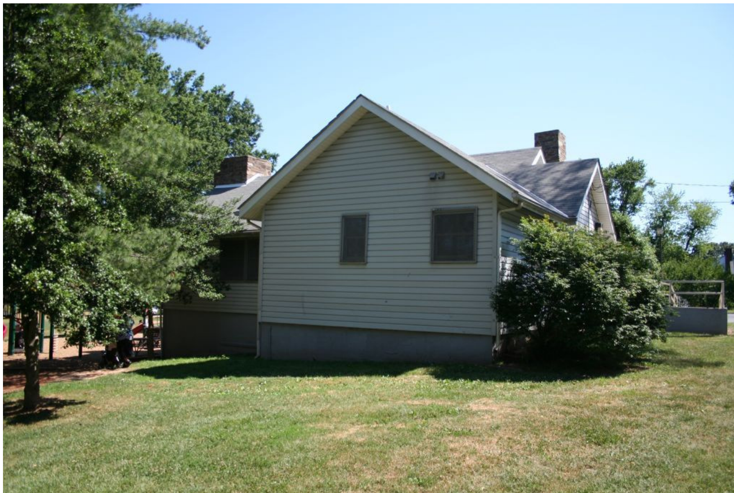
Figure 11. View of Pinecrest Recreation Building, south elevation.
