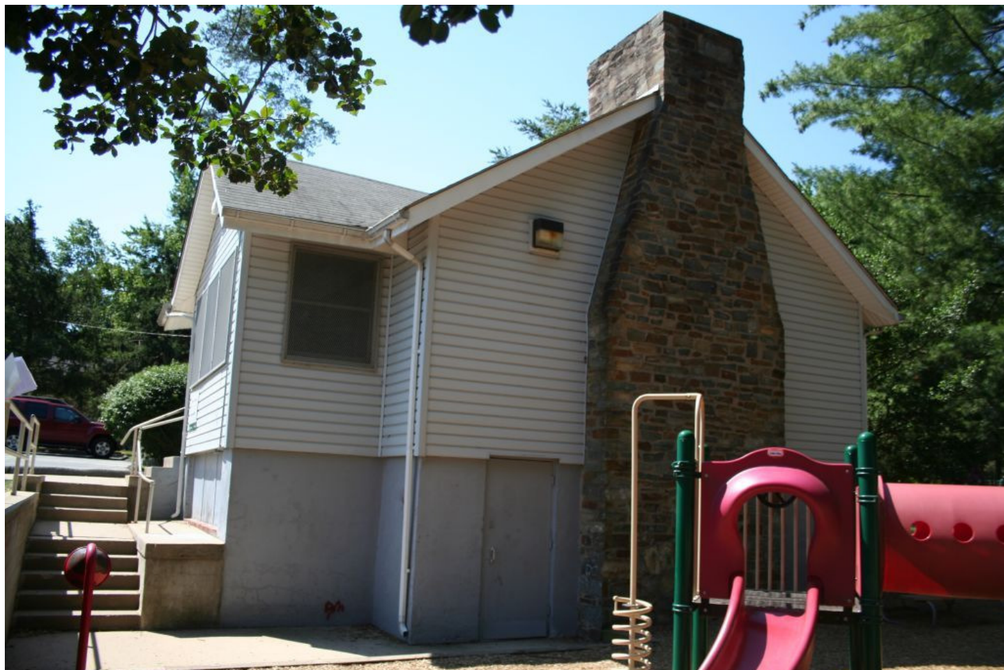
Figure 12. View of Pinecrest Recreation Building, west elevation.
