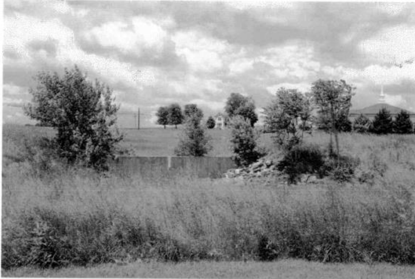
Tri-County Baptist Church storm water embankment overgrown with trees and vegetation
