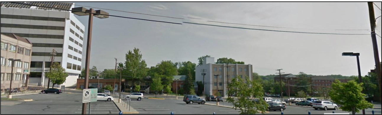
Street level view of frontage along Blueridge Avenue viewed from across Parking Lot 14
