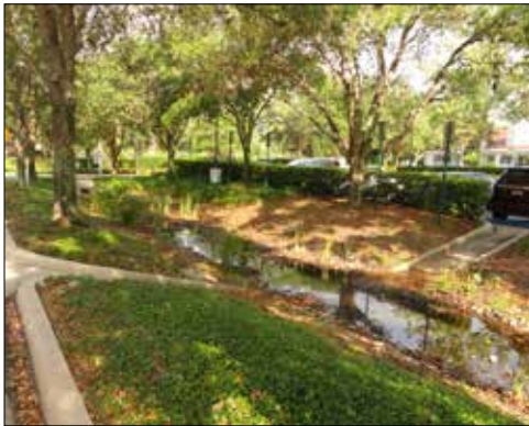
Orlando, FL: Landscaped islands in a parking lot provide an area for stormwater collection.
