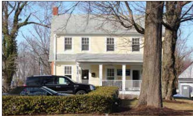
1001 Olney Sandy Spring Road: The former residence immediately west of the Holly Cottage is an example of a Colonial Revival building with a Dutch influence. It has five bays with a gambrel roof with projecting dormer windows.
