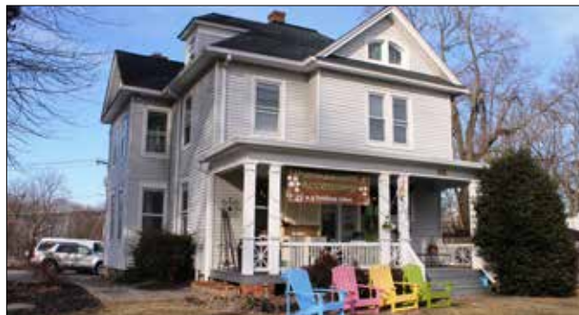
Holly Cottage: The former residence is a two-story Queen Anne-style building with a hipped roof and a cross gable. There is a small, double rounded window in the gabled end of the roof.
