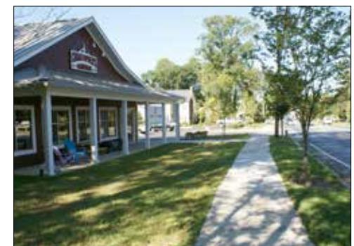
Existing buildings within the Sandy Spring Rural Village
