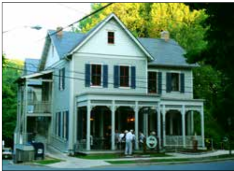
Garrett Park, MD: Adaptive reuse of an existing building into a retail use.
