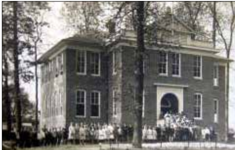
Sherwood School (demolished) Source: The Sandy Spring Museum
