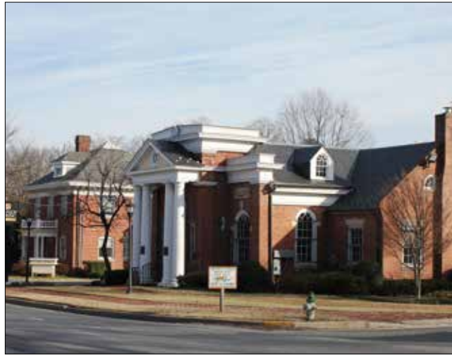
Sandy Spring National Bank (foreground) and the Montgomery Mutual Insurance Company (background): Both buildings are examples of Colonial Revival architecture. The bank is one-story high and three bays wide with a center gabled roof hidden behind a front façade. The insurance building is a two-story, three bay by two bay brick structure with a low bracketed, overhanging hipped roof with a pronounced, bracketed cornice. There is a large single bay hipped dormer within the roof along the front of the building.
