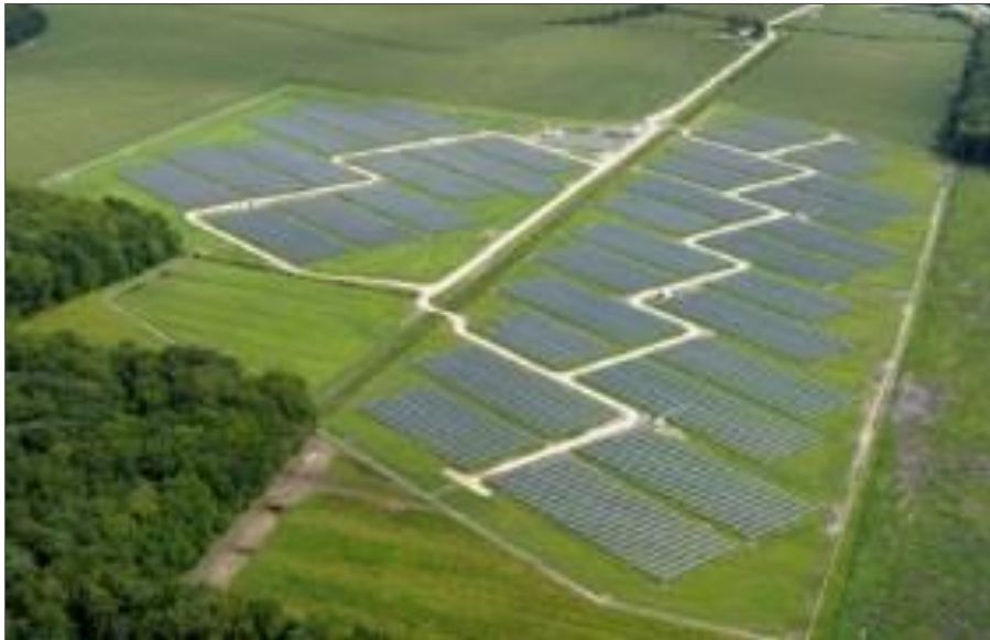
Above - Ground mounted solar array, Dover Delaware
