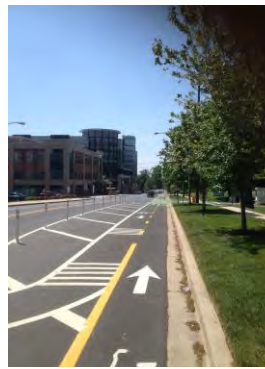
Woodglen Drive separated bike lane
