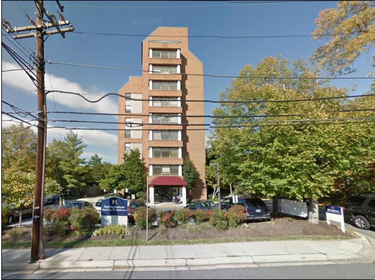
Figure 2-Existing Site, View from Battery Lane
