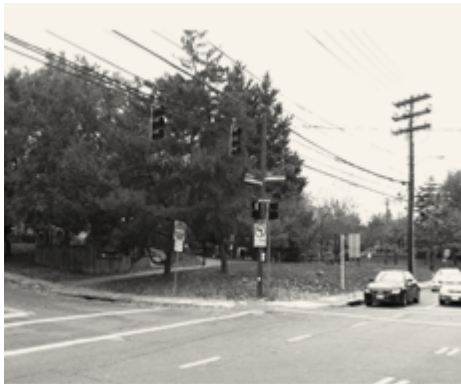
Existing Entry View from southeast
