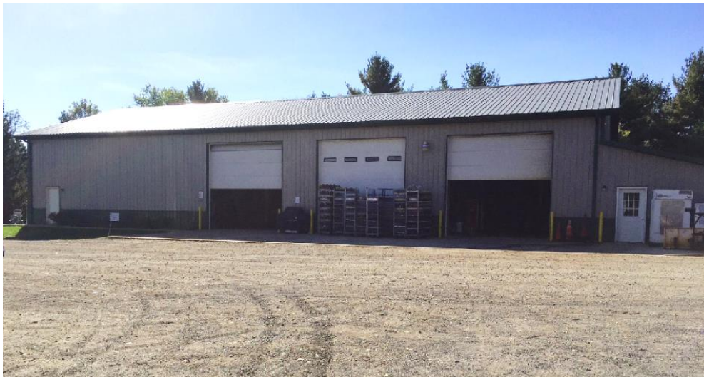
Figure 5: Pole Barn A
