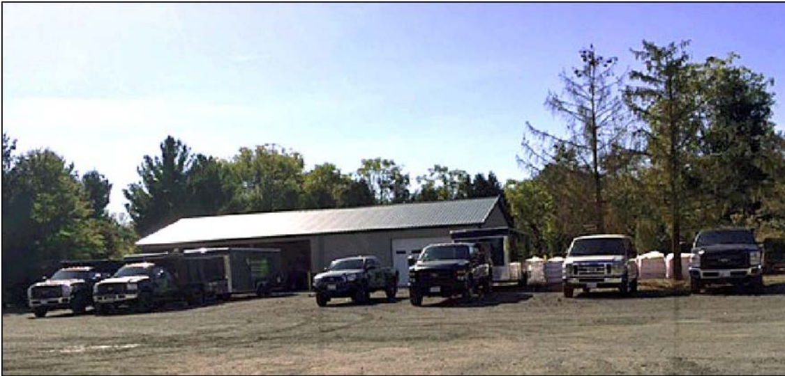
Figure 6: Pole Barn B
