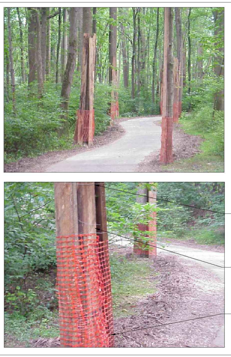
TREE PLANKING DETAIL N.T.S.
