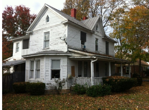
Figure 6: Farm House View from Driveway
