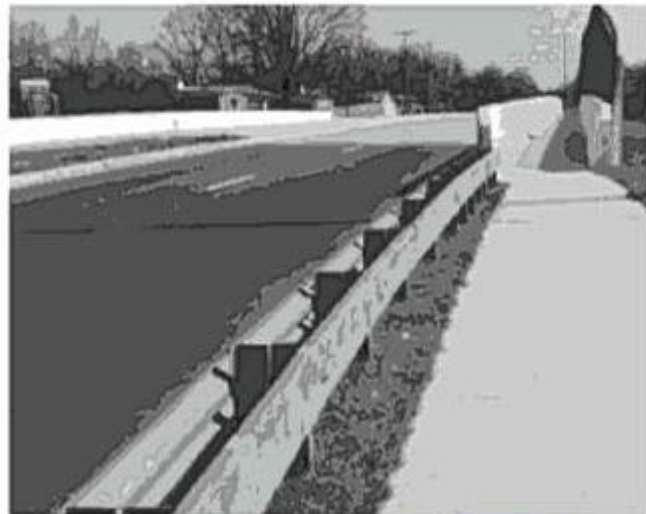
Figure 5-5. Protective rail on the backside of a guardrail adjacent to the sidewalk.
