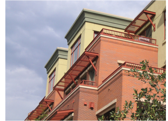
Sustainable and attractive buildings
