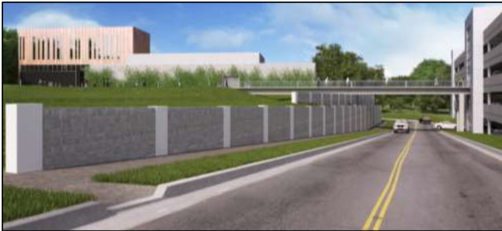
View of Bridge from the East
