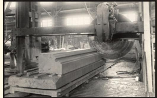
*Large stone-cutting machine at Fuller Plant*
