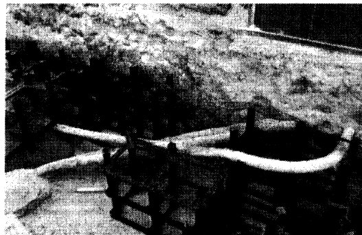
Silva Cells accommodate new and existing utilities.
