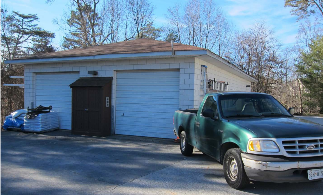
Maintenance building (to be removed—functions will be incorporated into new gym)
