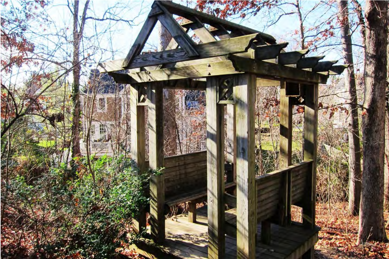
Covered bench in easement area (to be removed)
