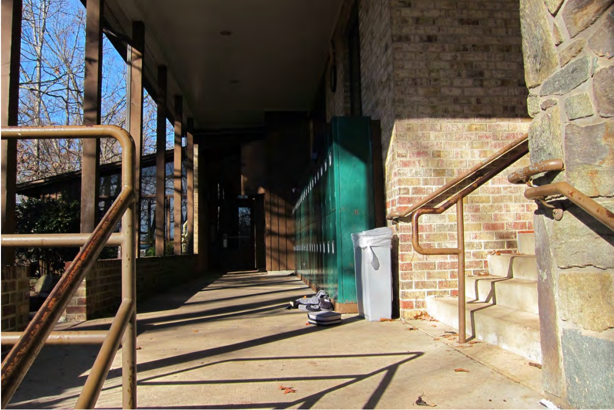
West side of middle school wing with outdoor lockers
