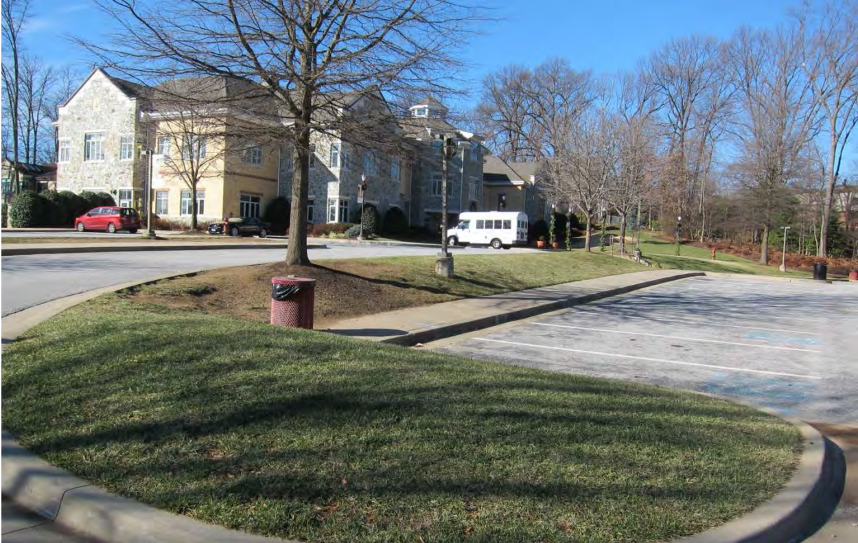
Main parking lot
