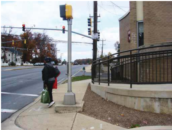
PROXIMITY OF BUILDING TO ROAD
