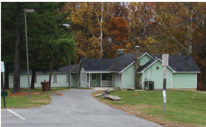
EXISTING RECREATION STRUCTURES
