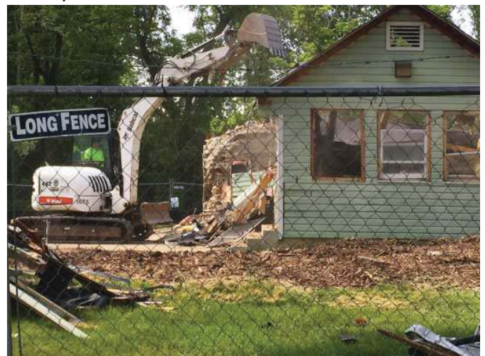
DEMOLITION OF RECREATION STRUCTURES
