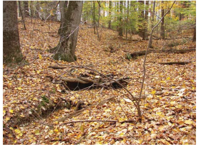
INTERMITTENT STREAM EROSION
