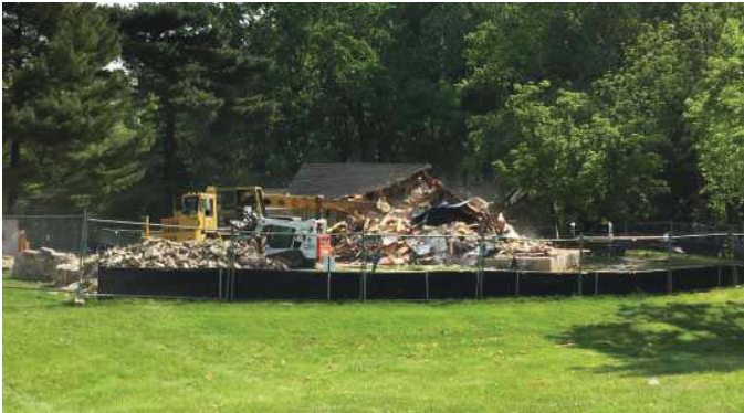
DEMOLITION OF RECREATION STRUCTURES
