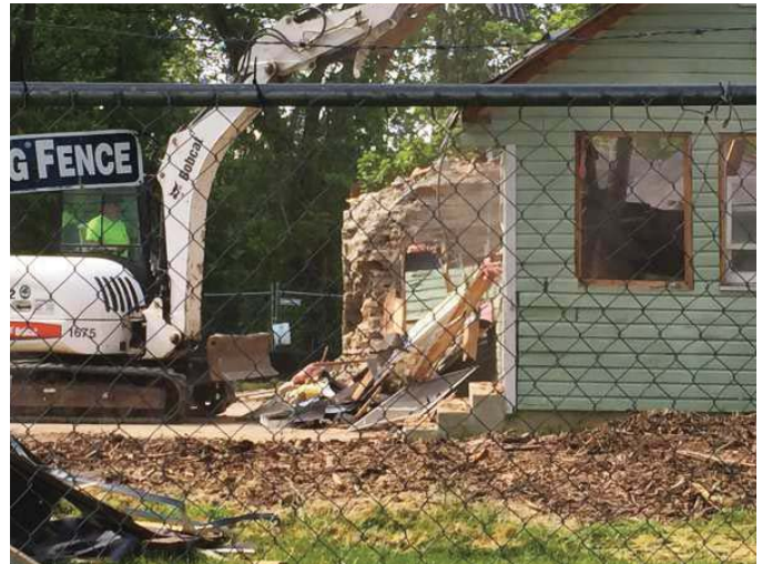
DEMOLITION OF PARK STRUCTURES
