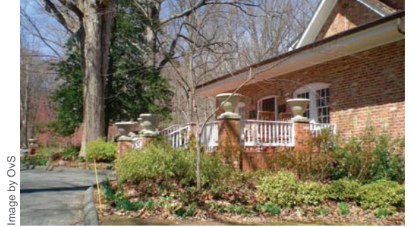
MANOR HOUSE (EXISTING)
