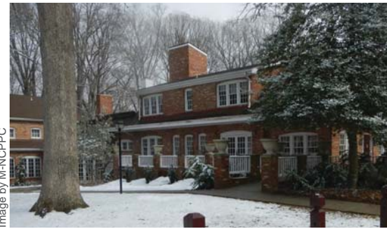
MANOR HOUSE (EXISTING)
