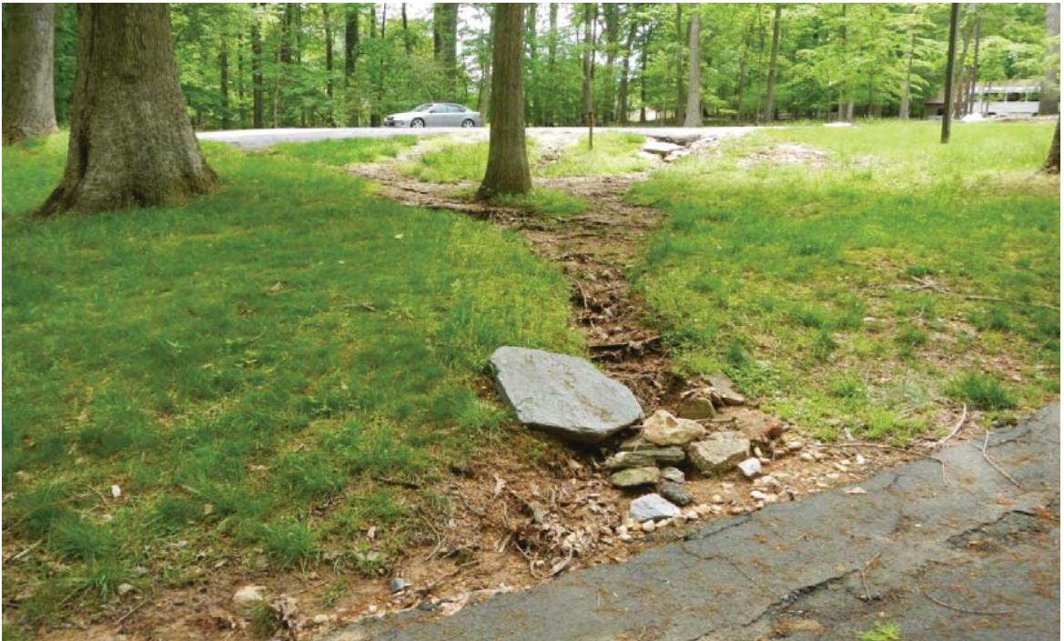
EROSION ON SLOPES (EXISTING)
