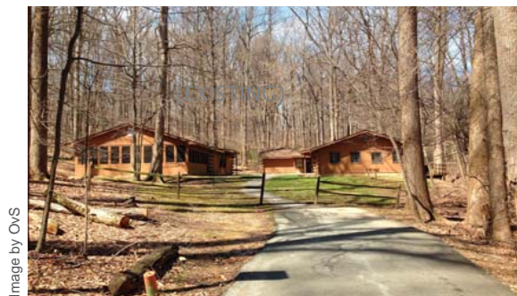
BUNK HOUSES (EXISTING)
