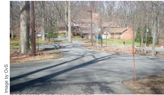
PARKING LOT (EXISTING)
