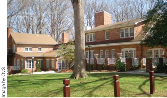
MANOR HOUSE (EXISTING)
