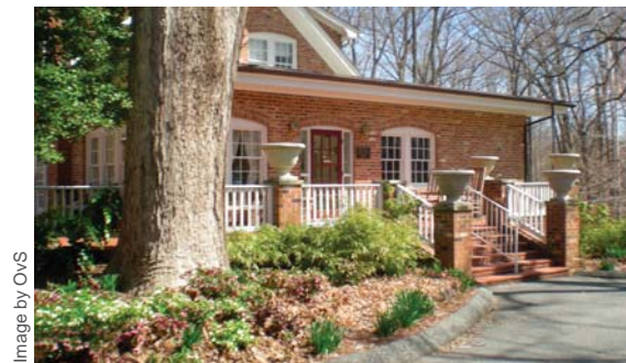
MANOR HOUSE (EXISTING)
