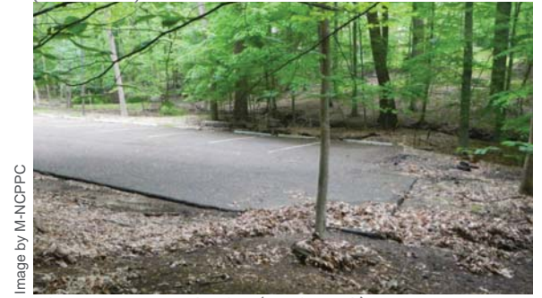
LOWER PARKING LOT (EXISTING)
