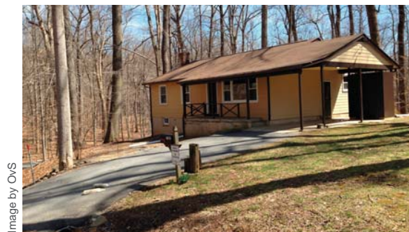
CARETAKER'S RESIDENCE (EXISTING)
