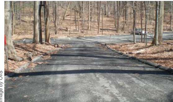
LOWER PARKING LOT (EXISTING)
