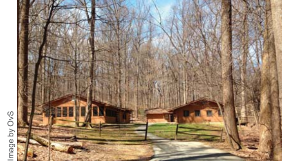
LOWER PARKING LOT TO BUNK HOUSES (EXISTING)
