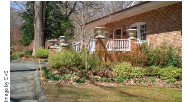
MANOR HOUSE (EXISTING)
