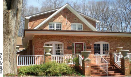
MANOR HOUSE (EXISTING)
