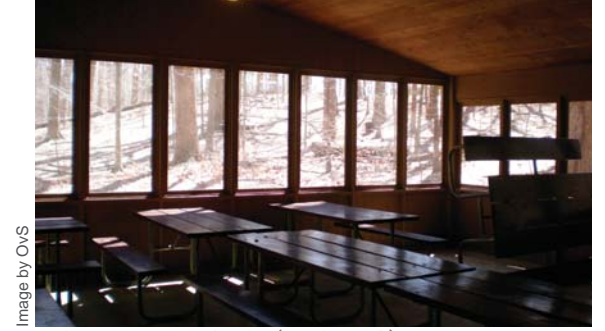
INSIDE BUNK HOUSE (EXISTING)
