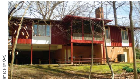
SKYVIEW LODGE (EXISTING)
