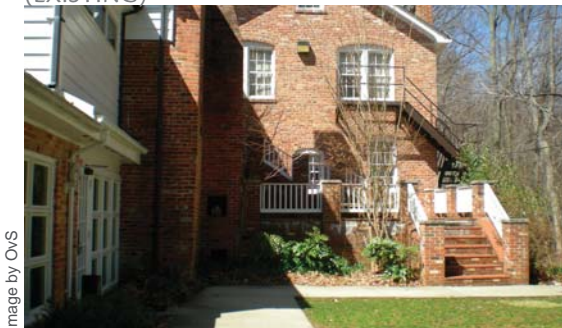
BACK OF MANOR HOUSE (EXISTING)
