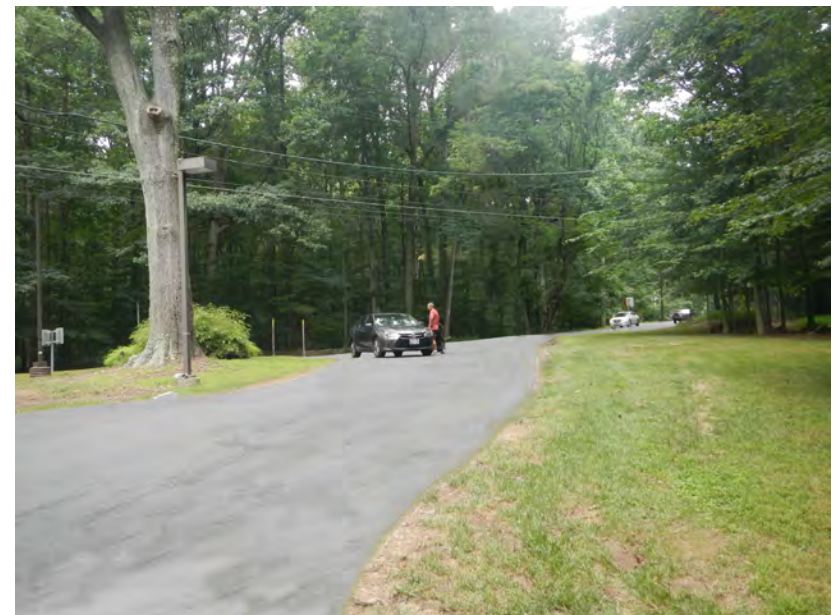
Widened two-way entry/exit drive. Note the removal of the tree on the right and the brick pillar on the left.
