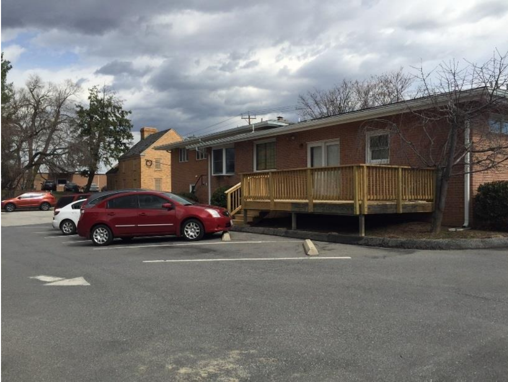
Figure 5: View of the rear of building (facing north)
