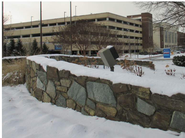
Existing walls in the Life Sciences Center
