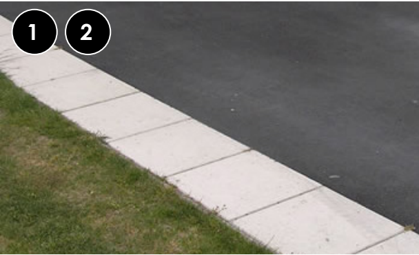
Paver edging with asphalt path
