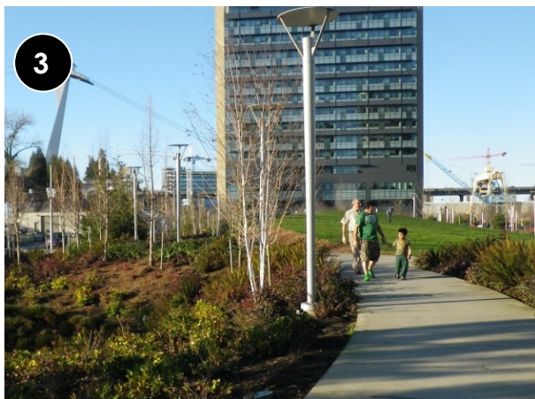
Planted bioretention areas
