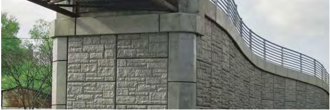
Figure 17: Ashlar Stone Abutment Example
