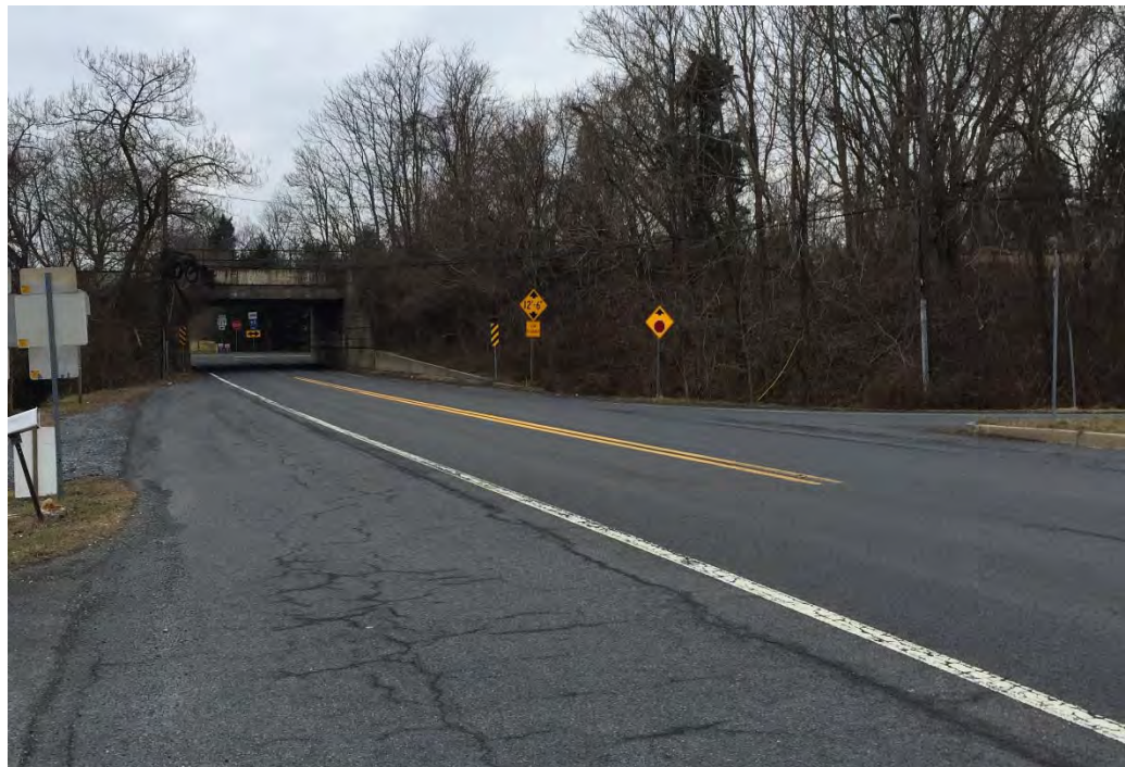
Figure 4: MD 117 Approaching Rail Bridge (looking south)
