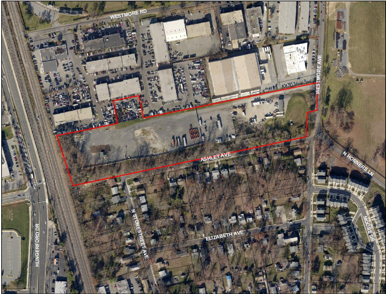
Image 2: Site Aerial View
