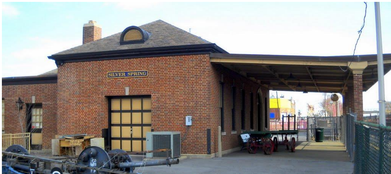
View looking south toward the Silver Spring B&O Station.
