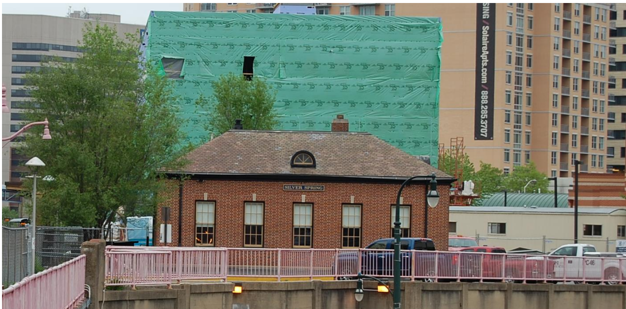
View looking northwest of the historic Silver Spring B&O Railroad Station with the new Progress Place in the background wrapped in green Tyvek.
