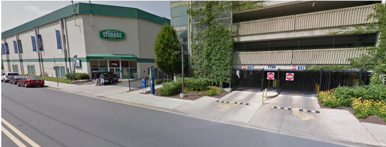
Driveways at Extra Space Storage (left) and the Montgomery College Parking Garage (right)
