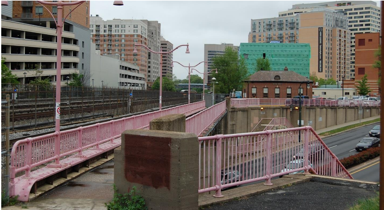
A view of the existing CSXT/WMATA tracks looking northwest toward the B&O Station.
