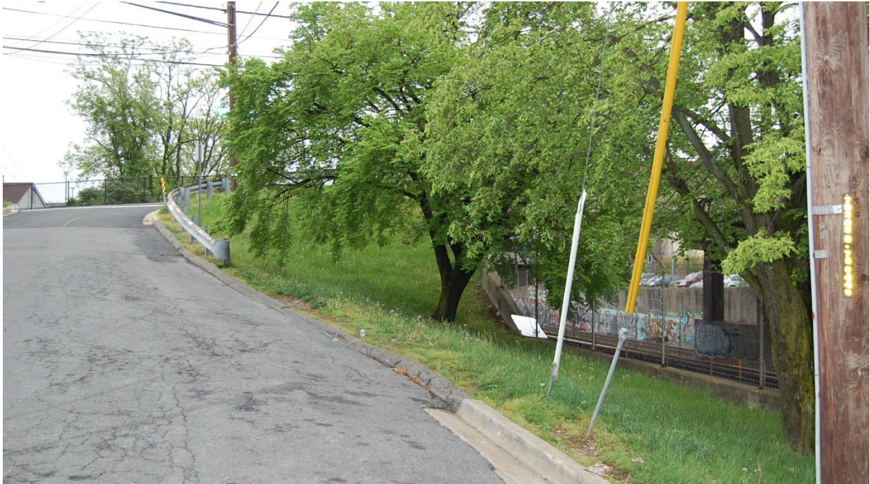
View looking southeast . The proposed location of the new underpass will be located beneath Burlington Avenue in the grassy area between Selim Road (left) and the CSXT/WMATA tracks (right).
