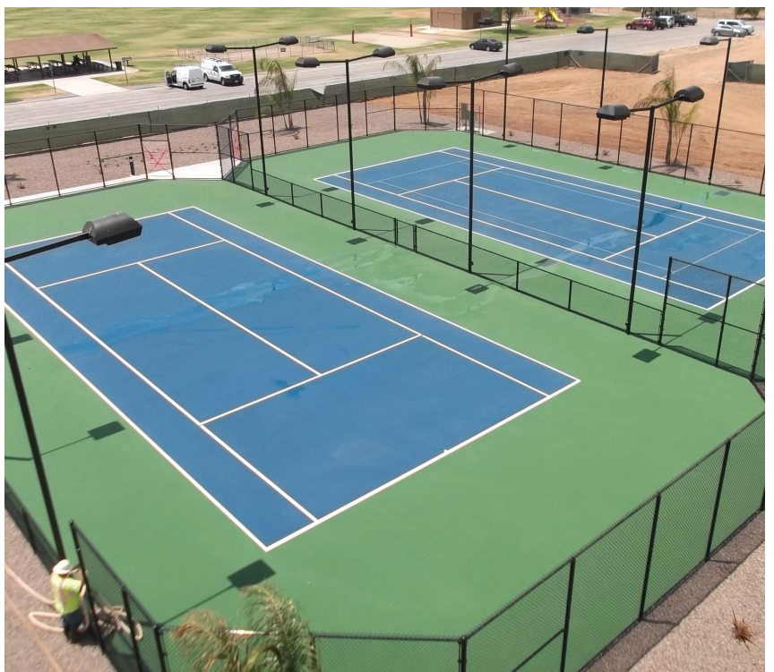
Public tennis courts, Miramar, FL
