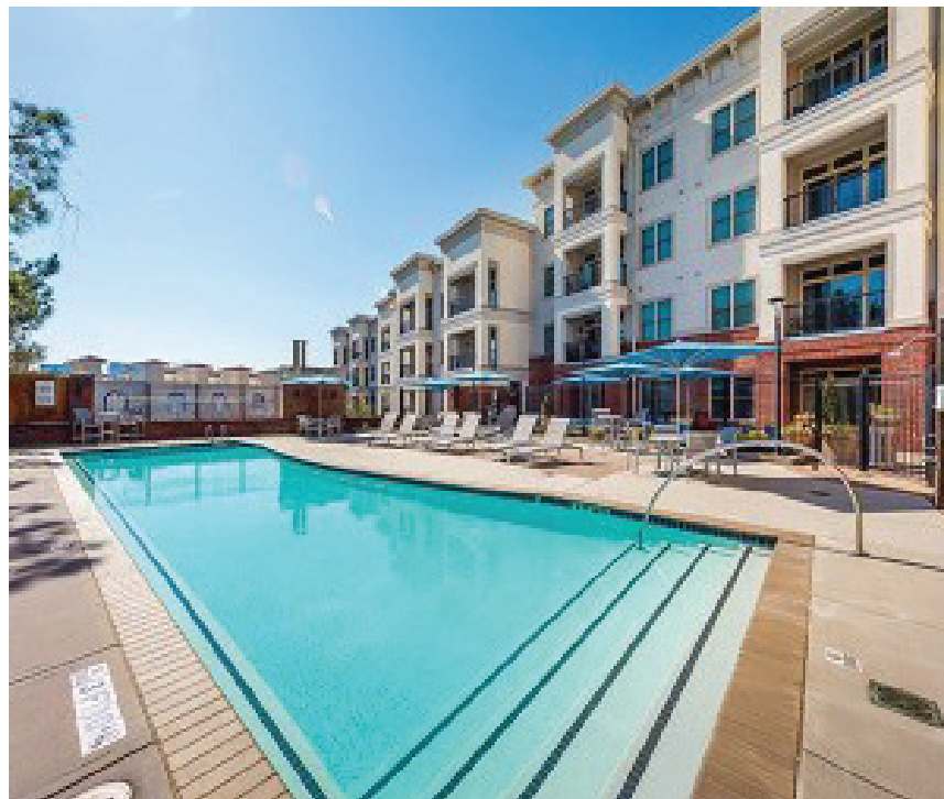
Outdoor pool, Tremont Apartment Homes, Atlanta, GA
