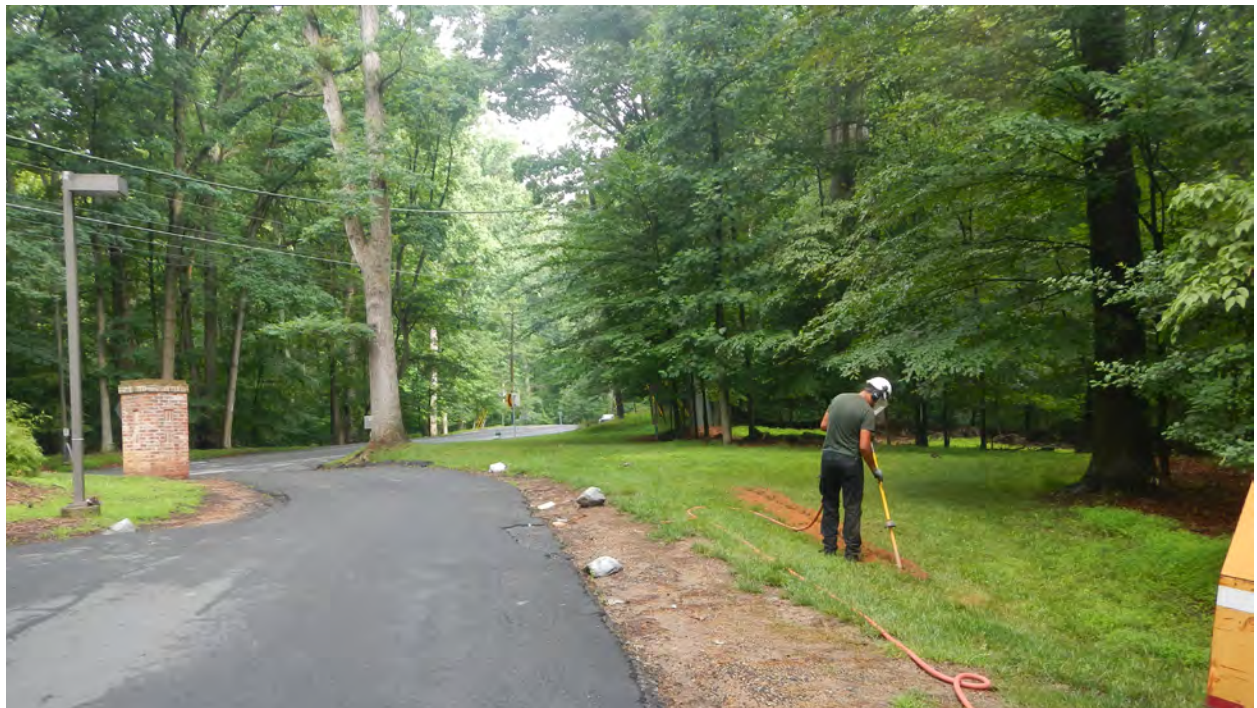
Air spade root investigation operations at the park's vehicular entrance. While investigations within the compacted areas alongside the driveway (where no grass is growing) revealed minimal tree roots, an abundance of tree roots were discovered in the lawn and mulched areas along the park's frontage with MacArthur Boulevard.
