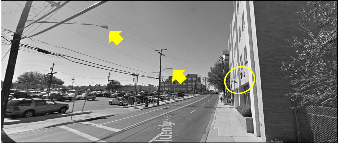
Photograph of Blueridge Avenue looking west highlighting existing lighting fixtures to remain
