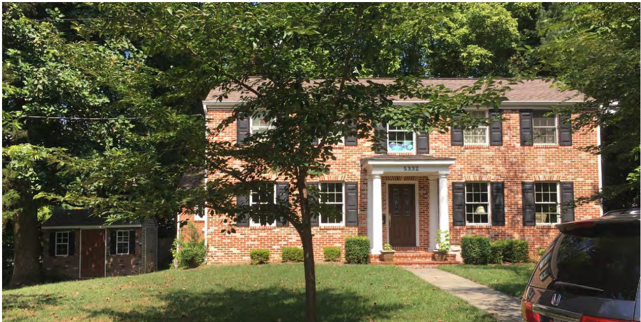
Figure 3: Photo of 5332 Allandale Road (looking northwest)
