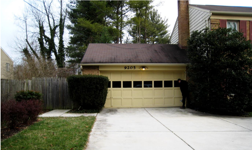
Figure 11: Existing Driveway Adjacent to Northern Property Line
