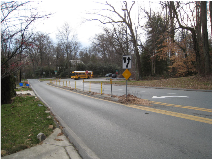
Figure 3: Raised median with traffic flex poles on Fernwood Road (looking south from the site)
