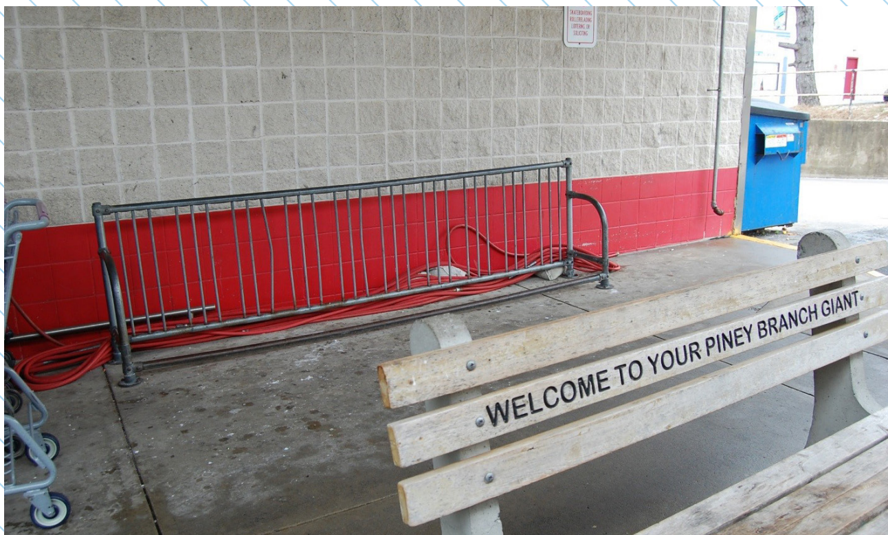
Improperly installed bicycle racks limit use
