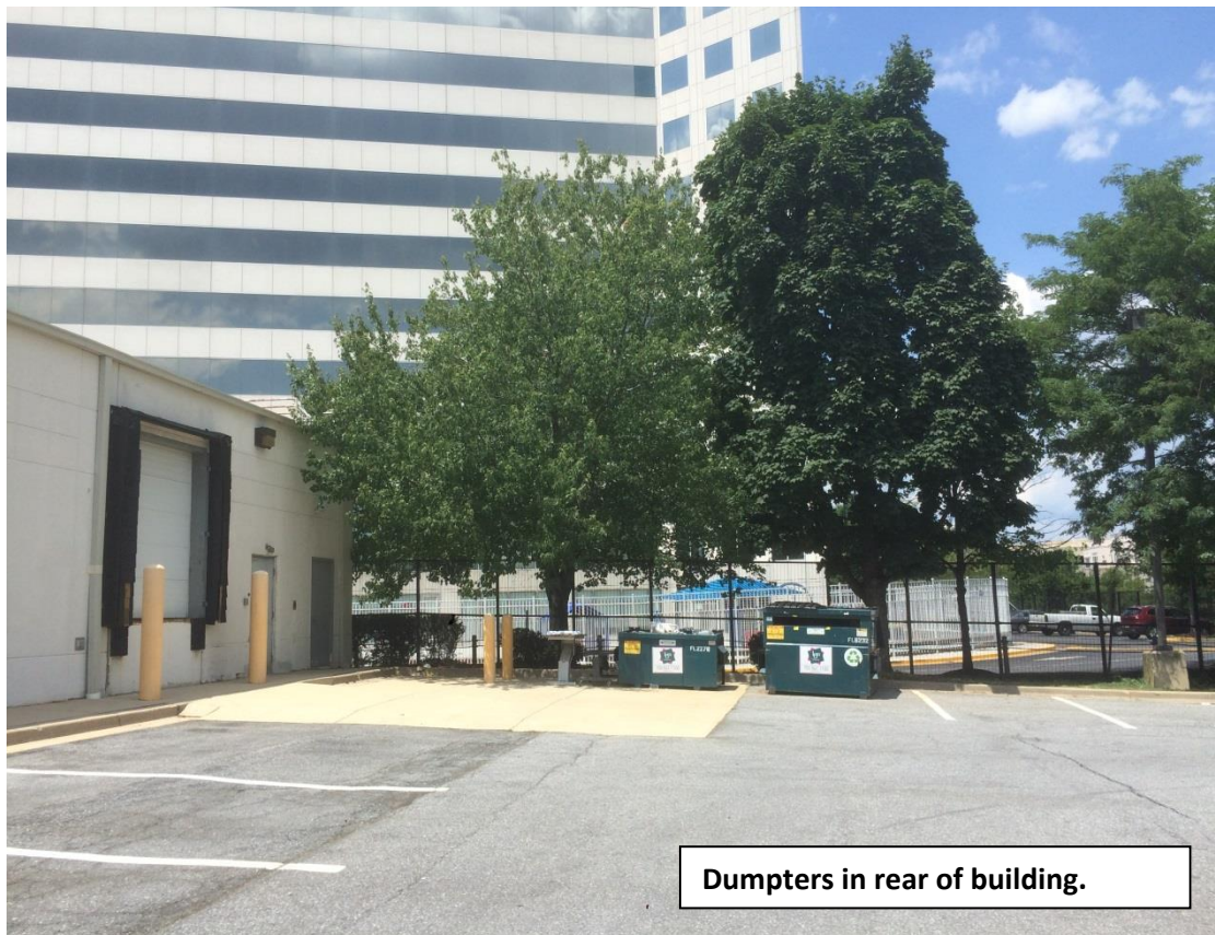
Rear of building facing northwest.
