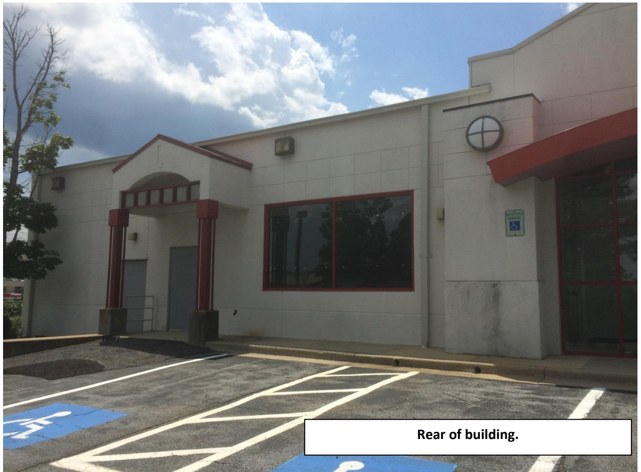
Rear of unit.
