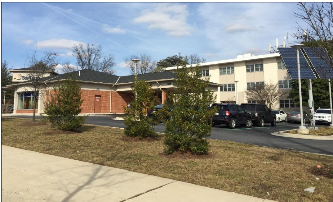
Figure 3: View from Old Georgetown Road (facing northeast)
