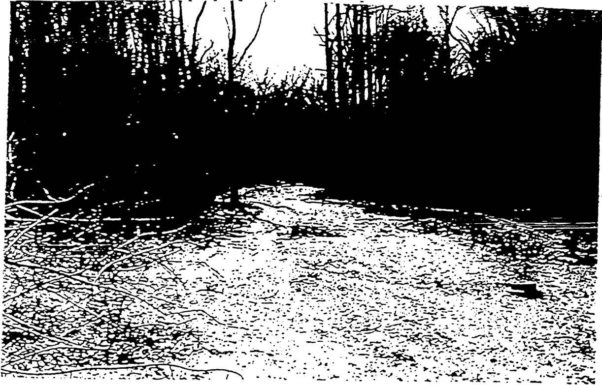
CLEARED WSSC SEWER RIGHT-OF-WAY, LITTLE SENECA CREEK GREENWAY
