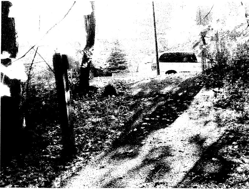
Photo – 1. Existing steep slope at access point
